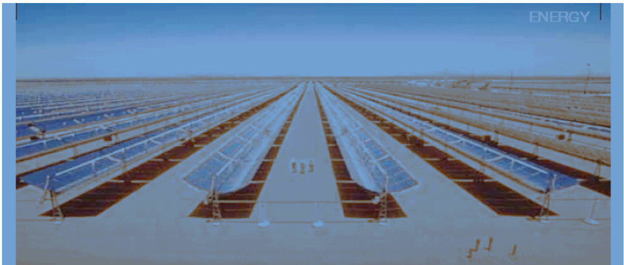
Figure 3. Parabolic trough concentrating solar collectors. [3]
