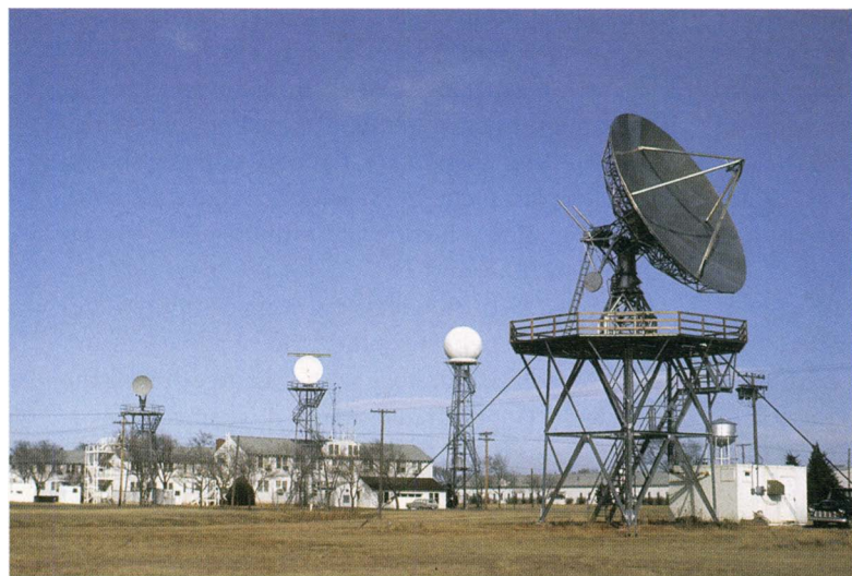
FIG. 5. (right) Norman 10-cm pulsed Doppler radar antenna and pedestal on an open tower with the transmitter in the building at the base (1969). (The decommissioned antenna and pedestal are now on permanent display at ground level on the same site.) The open tower was chosen as a cost-savings measure, but it proved to be unsatisfactory. So, the antenna and pedestal were subsequently moved to the permanent building shown in Fig. 6. The radar to the left of the tower was NSSL's WSR-57 research surveillance radar. The other two radars in the left part of the picture were used for aircraft tracking as part of Project Rough Rider. The two-story former Navy barracks building behind the three radars housed NSSL's Weather Radar Laboratory and then NSSL from 1962 through 1972. [NSSL photo.]
