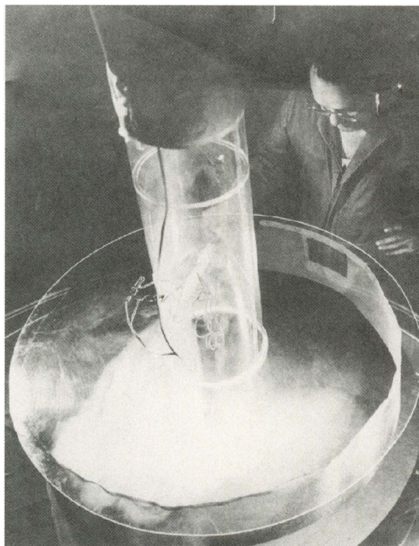
FIG. 7. Neil Ward monitoring the development of a tornado vortex in a small version of his famous tornado chamber. [Photo copyright of History of Science Collections, University of Oklahoma Libraries.]
