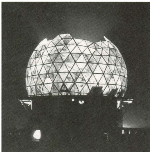
FIG. 9. Nighttime view of the radome on NSSL's Cimarron Doppler radar building being assembled by the Oklahoma Air National Guard in 1973. [NSSL photo by Charles Clark.]
